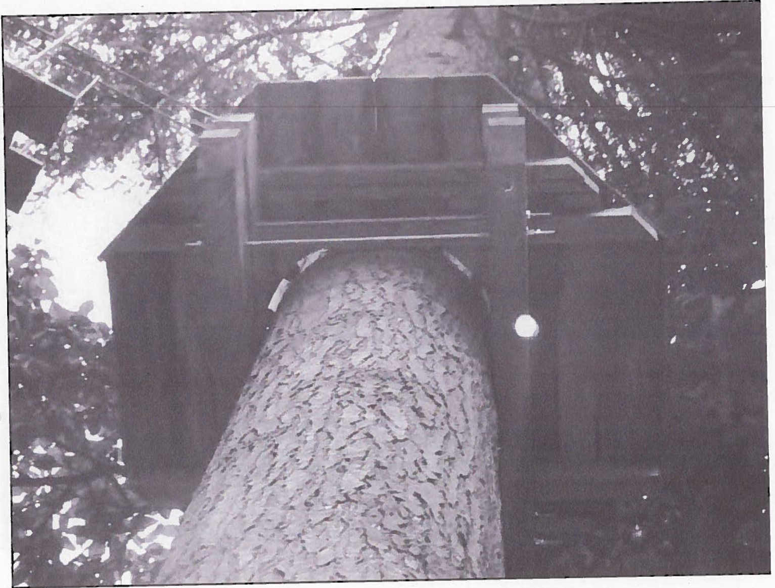
Example of Brace and Platform Construction
